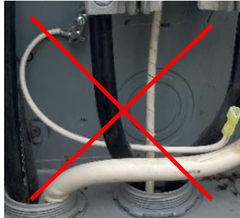
Figure 1: Neutral lead from meter base plug-in transfer device is connected to meter base ground terminal
