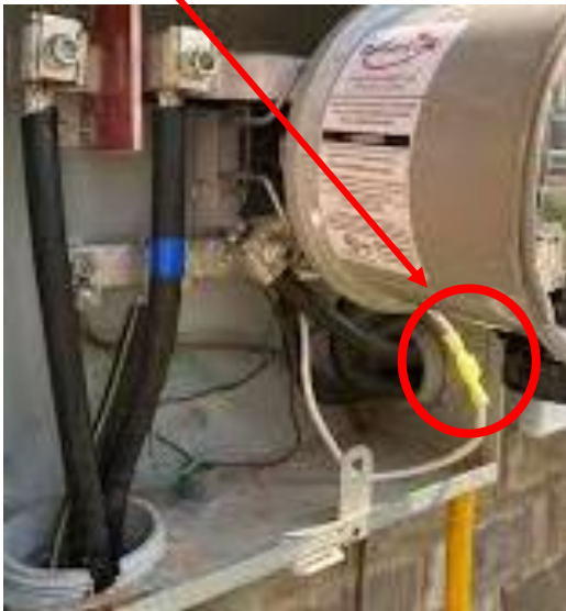
Figure 4: Spade type connection to neutral Figure 5: Plug-in device with use of bracket
