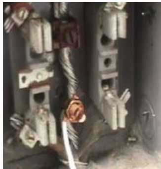
Figure 3: Compliant neutral connection to meter base plug-in transfer device
