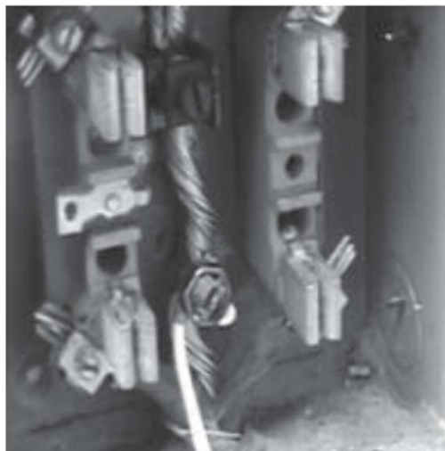
Step 2b Split-nut Installation
