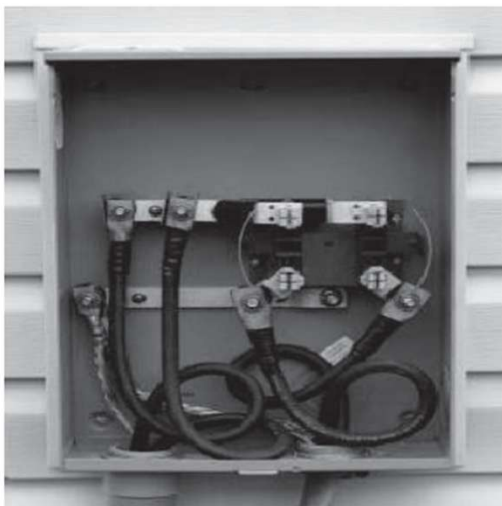
Step 2a Hi-Lug Installation
