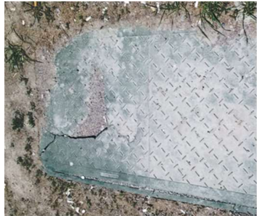
Utility service cover that has been damaged.
