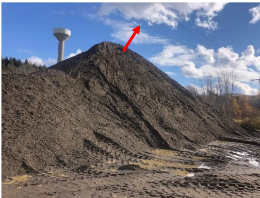
Picture 1: Stockpile of sand under the overhead powerlines
