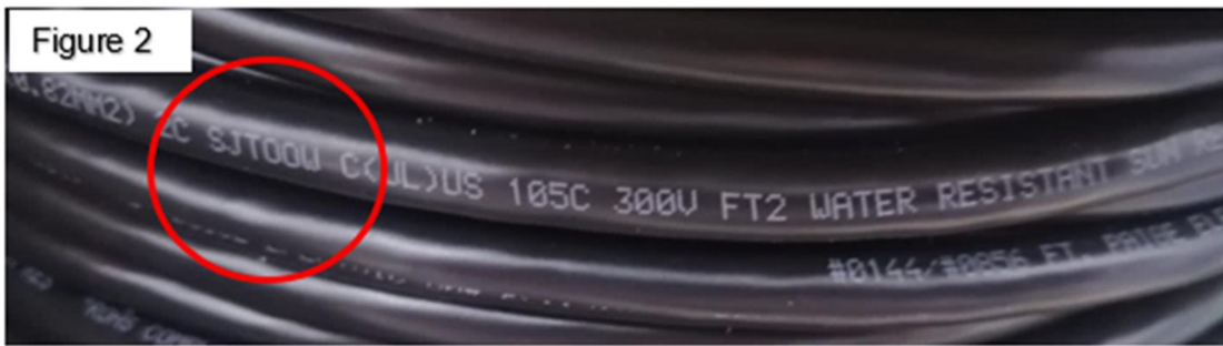
Figure 2: Compliant cable (SJTOW marking)
