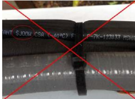
Photo 3 - SJOOW flexible cord used for interconnection wiring of a split system
