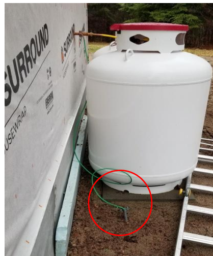
Diagram 12 – LP line connected to separate grounding electrode is not permitted
