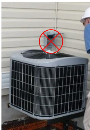
Photo 4 – 1 metre of working space required
