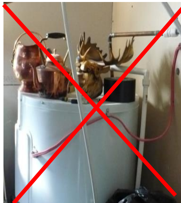
Photo 2 - NMSC not protected by location
