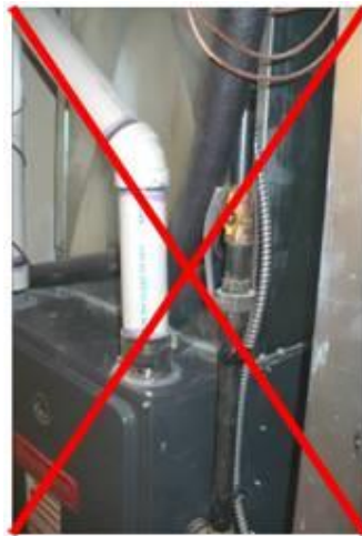
Photo 1 – Use of electrical tape not acceptable for securing armoured cable to gas pipe or other support
