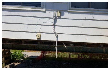
Picture 2: Example of breaking of the ground wire and exposed branch wiring
