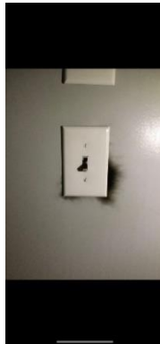
Picture 1, Damage due to Arcing
