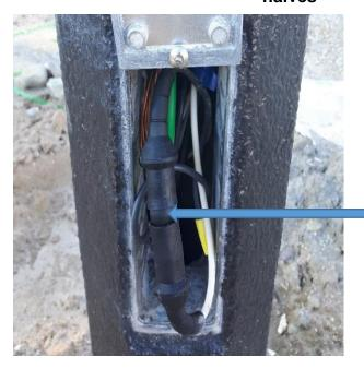
Wide Gap between fuse holder halves when assembled
