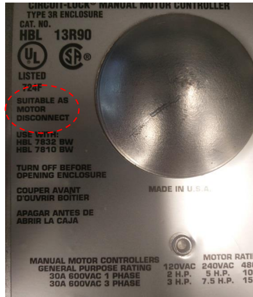
Photo F1 – Manual Motor Controller marked as “Suitable as Motor Disconnect”
