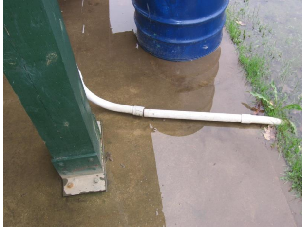
Photo F2 – Improperly protected conduit (Damaged)
