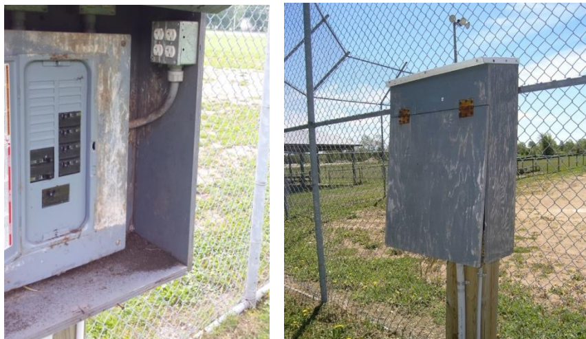
Photo F3 – Accessible and Deteriorated Enclosure
