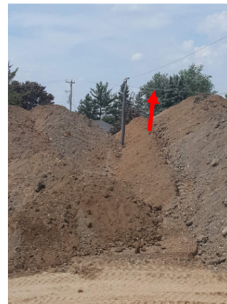
Picture 1: Stockpile of sand under the overhead powerlines
