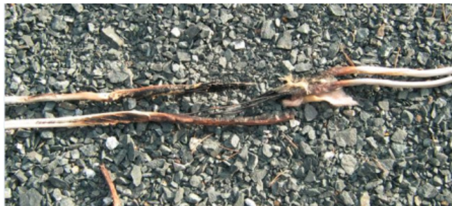
Photo F1 – Electrical equipment failure
