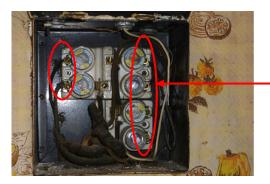
Many of these older electrical fuse panels may not provide adequate shock protection for persons replacing fuses. Persons are exposed to energized connections and conductors when accessing the fuses.
