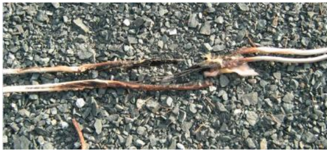
Photo F1 – Electrical equipment failure
