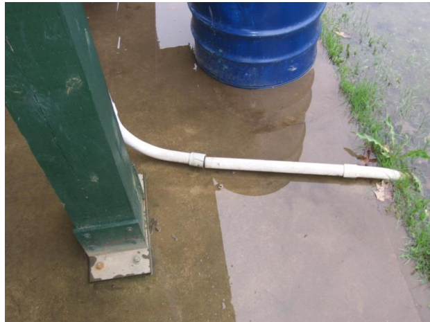
Photo F2 – Improperly protected conduit (Damaged)
