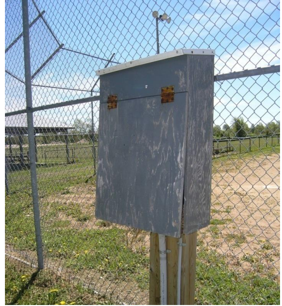
Photo F3 – Accessible and Deteriorated Enclosure
