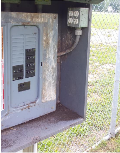
Photo F3 – Accessible and Deteriorated Enclosure
