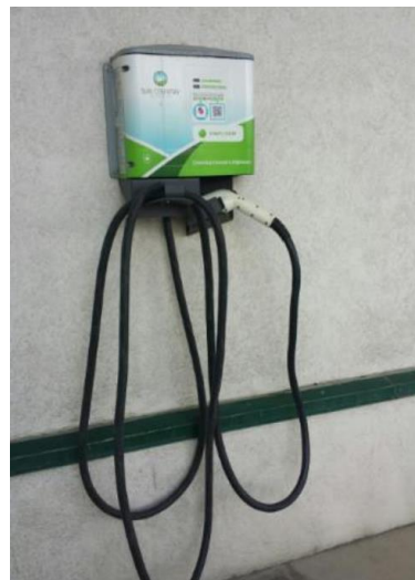
Photo B4 – EVSE protected by height
