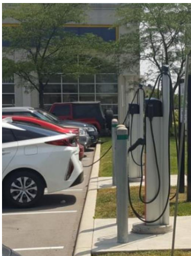
Photo B3 – EVSE protected by bollards
