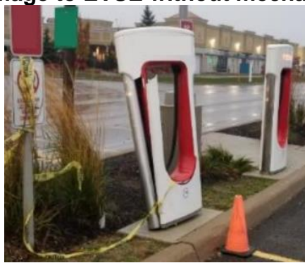
Photo B1 – Damage to EVSE without mechanical protection
