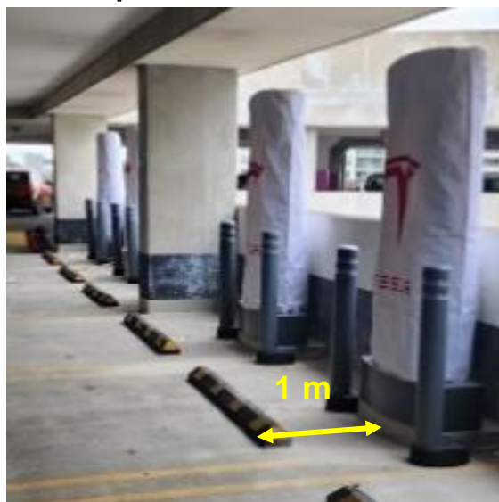
Photo B3 – EVSE protected by curb stop
