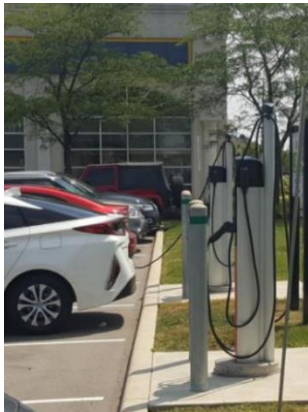
Photo B2 – EVSE protected by bollards
