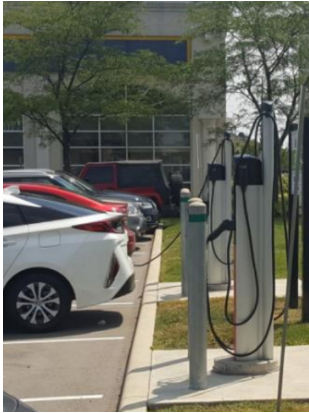
Photo B3 – EVSE protected by bollards by height
