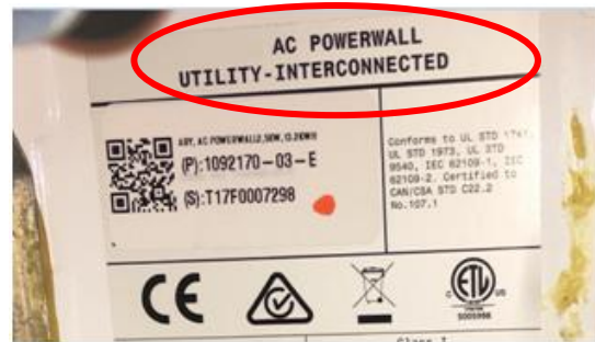
Photo B1 - Example of self-contained energy storage system and nameplate
