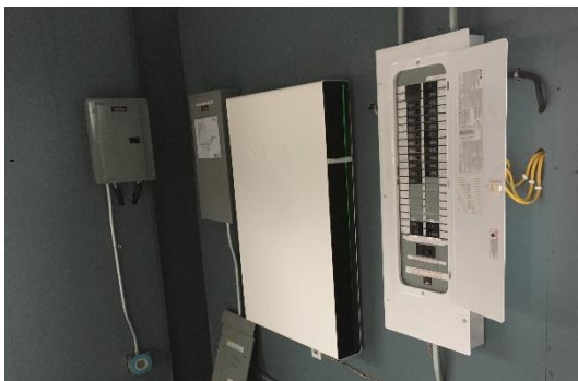
Photo B1 - Example of self-contained energy storage system and nameplate
