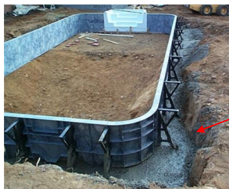
Photo B1 – Poured concrete for structural support
