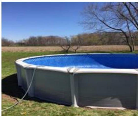
Photo B3 – Above ground pool with non-conductive supports
