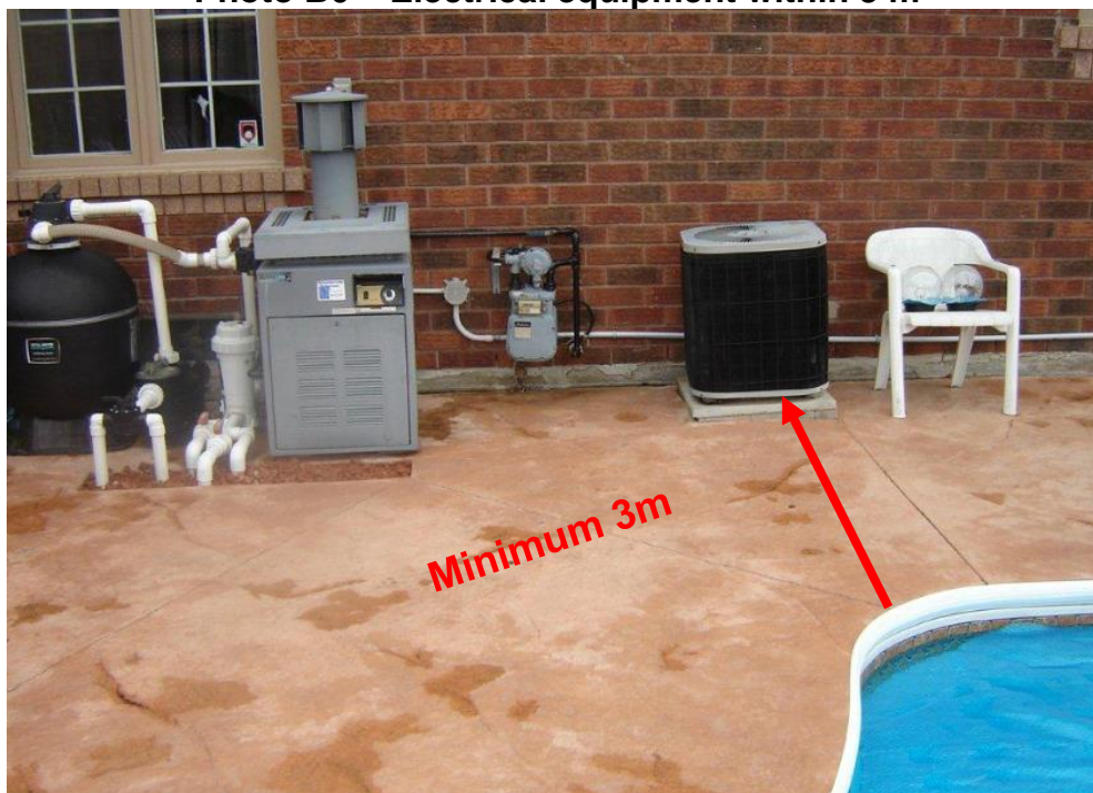
Photo B6 – Electrical equipment within 3 m
