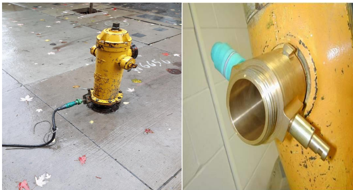
Photo B7- Example of hydrant grounding
