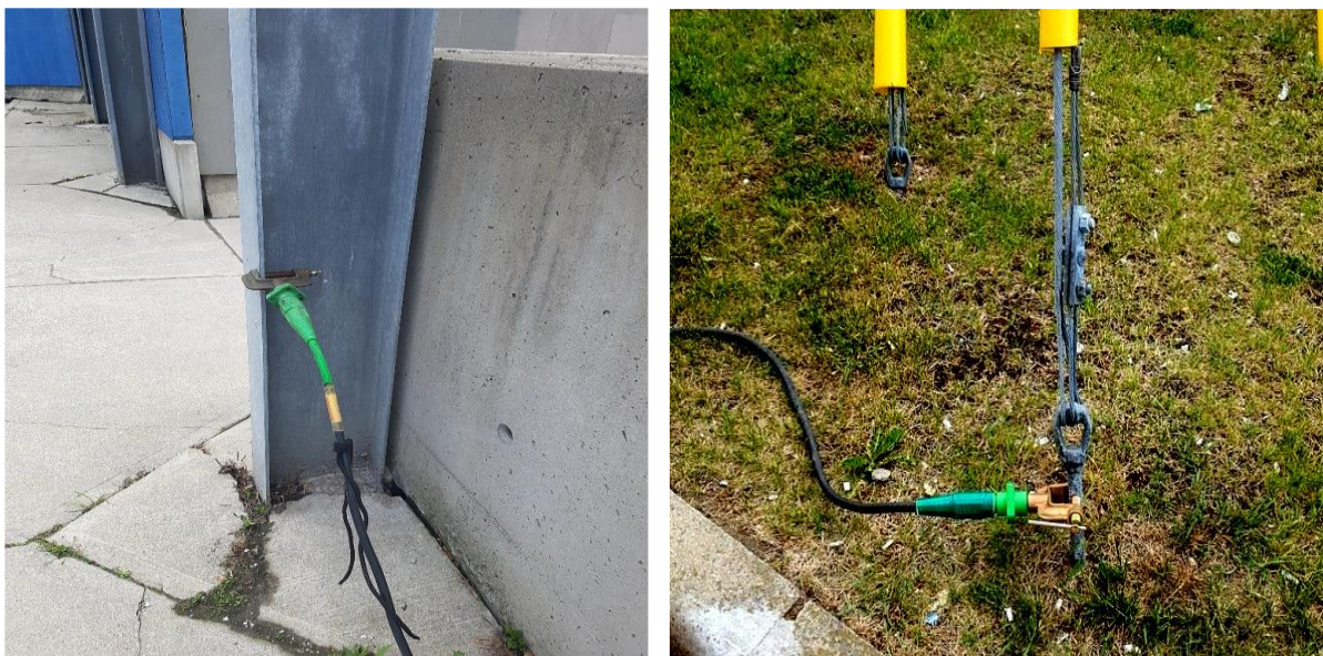
Photo B6- Example of acceptable in-situ grounding
