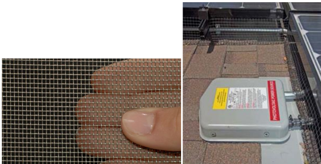
Photo B4 – Examples of acceptable screening for protection against rodents
