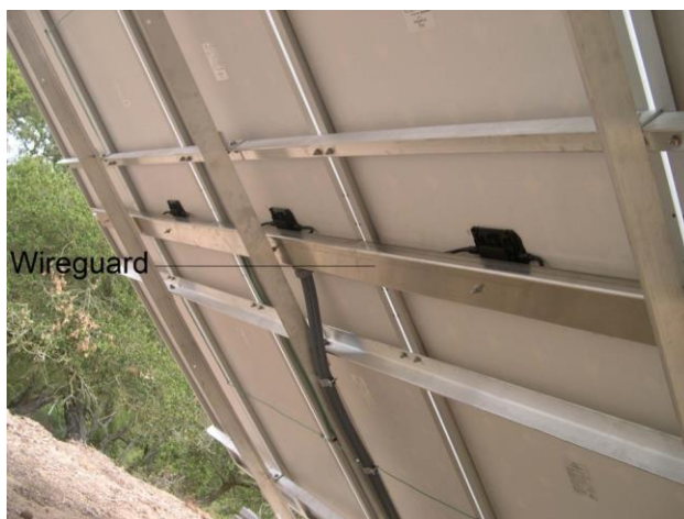
Photo B6 – example of using physical barrier around wiring
