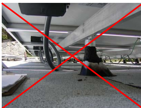
Photo B2 – Unacceptable cable support
