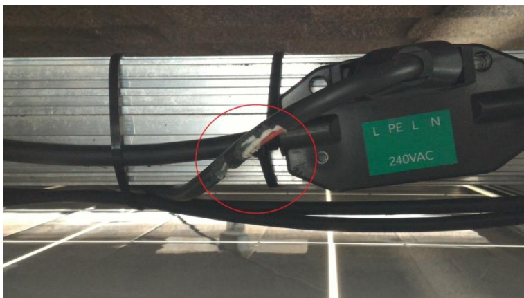
Photo B3 – Examples of rodent damage
