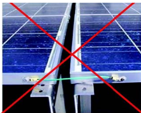
Photo B1 – Unacceptable bonding conductor connection
