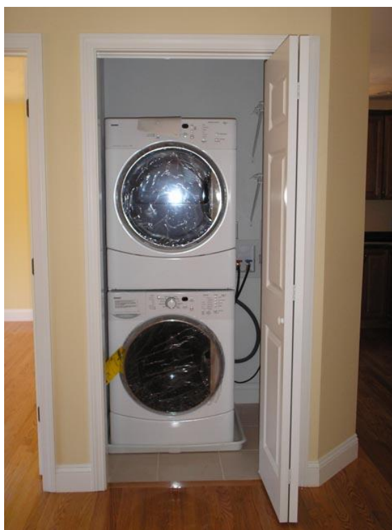
Photo B1 – Laundry closet
