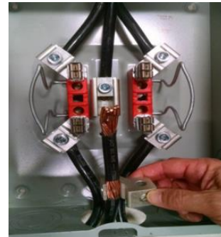
Photo B3 Compliant terminations Examples: split bolt, insulation piercing, separate connector
