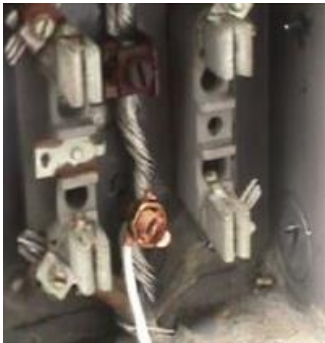
Photo B3 Compliant terminations Examples: split bolt, insulation piercing, separate connector
