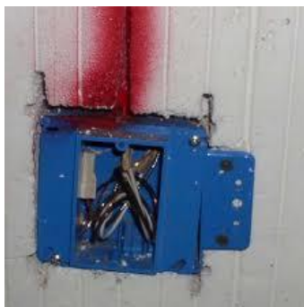
Photo B3 – Typical box installation in ICF form
