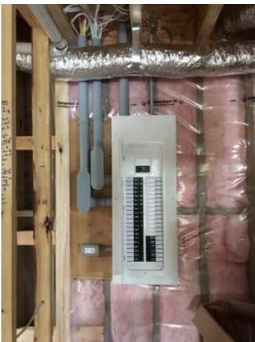
Photo B7 – Installation of in rigid PVC conduit to a panel
