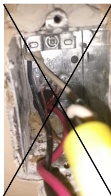
Photo B8 – A conductor that is not protected from sharp edges; non-Code compliant installation
