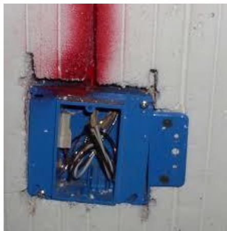
Photo B1 – Typical box installation in ICF form
