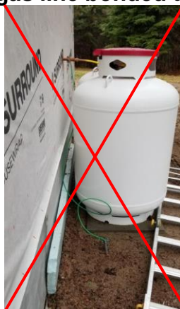
Photo B1 - Example of gas line bonded to a separate ground rod
