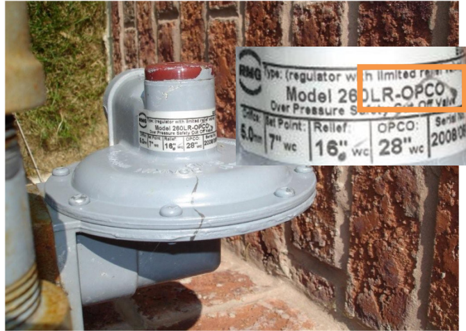
Photo B7 – Typical demarcation point between Gas Company and customer house line
