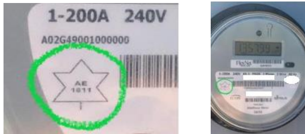
Photo B2 – Socket sub meter
