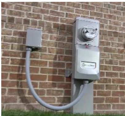
Photo B3 - Meter-mounted transfer switch
