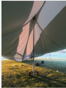
Figure 2: Dolly and tent cover obstructing view of overhead powerlines above
