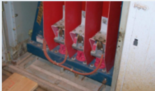
Figure 1: The contactor would be rolled out of the cell using the built-in rails in each compartment.
