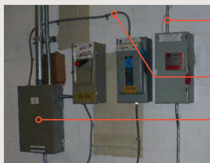
Figure 2: BX cable highlighted.
