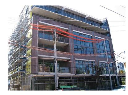
These covers are installed only as visual indicators and are a reminder to maintain safe distances. They do not provide electrical isolation and cannot be relied upon for preventing electrical shock. to perform such work, should never work within the minimum safe distances from overhead powerlines.
