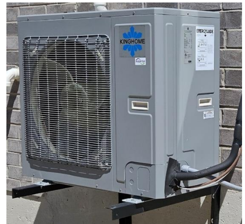
Heat pump for space heating/cooling
