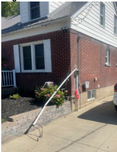
Damaged Overhead Service Conduit
