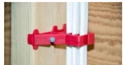
Approved cable stacker prevents fasteners from piercing NMSC
