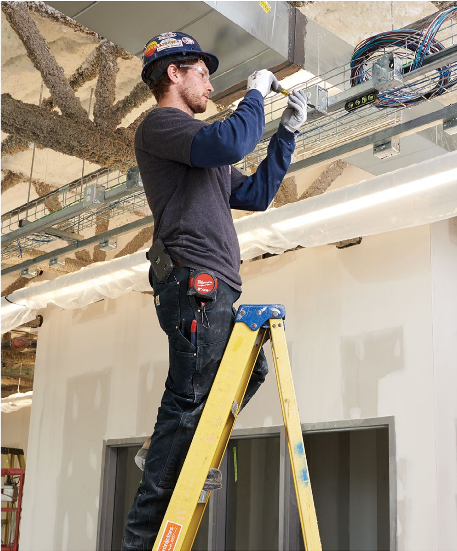
ESA worked together with industry, colleges and the Ministry of Labour to help electrical workers return home safely at the end of each day. Pictured: Corey Leadbetter, Birnie Electric.
