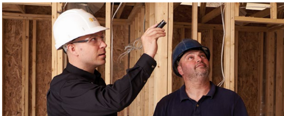
Inspector Matthew Munroe reviews a new electrical installation with Cosimo Pantaleo of Deerfield Electric to ensure it complies with the Ontario Electrical Safety Code.
